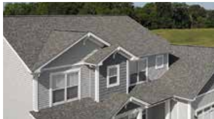
ROOFING AND VENTILATION
