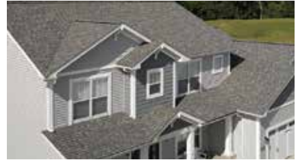
ROOFING AND VENTILATION
