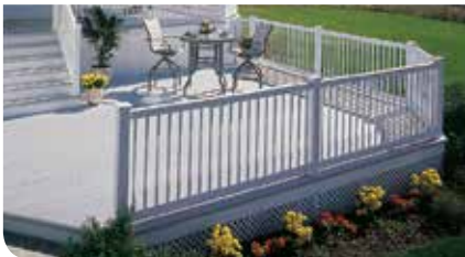
DECKING AND RAILING
