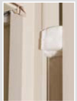
Foam blocks reduce air infiltration.
